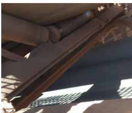
AFTER INSTALLATION ProTOUGH CONVEYOR BELT
