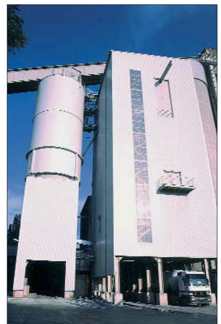
Building material mixing plant for up to 180t/h
