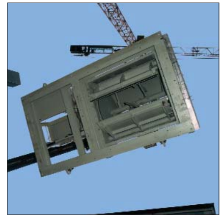
Assembly of a batch mixer with double-discharge flap system
