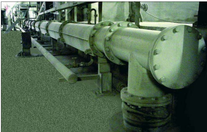
FLUIDCON transport system at Holcom Plant Lägerdorf for 230 t/h cement
